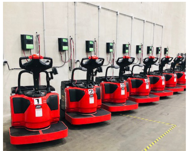
Figure 3: A power management system ensures that an electric lift truck fleet operates at full capacity.
